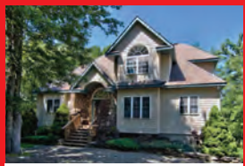
2932 South Fairway Drive $339,000
